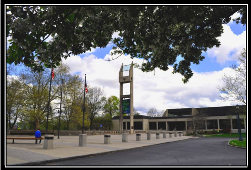
Municipal Services Center
