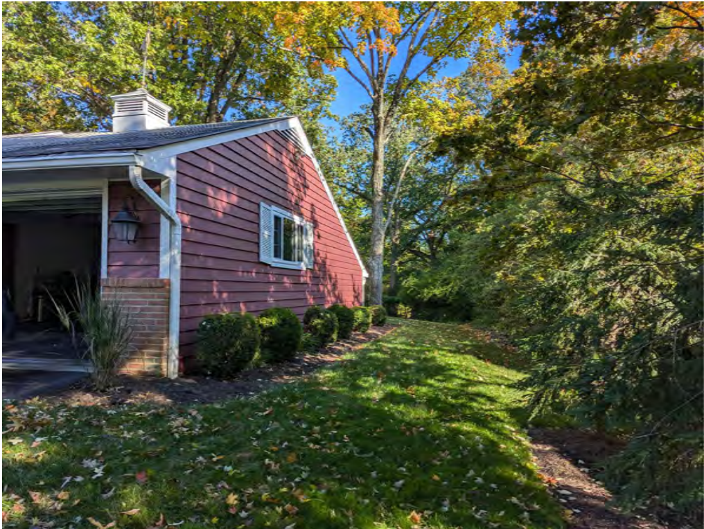
2 Existing South Side Elevation - Photo
