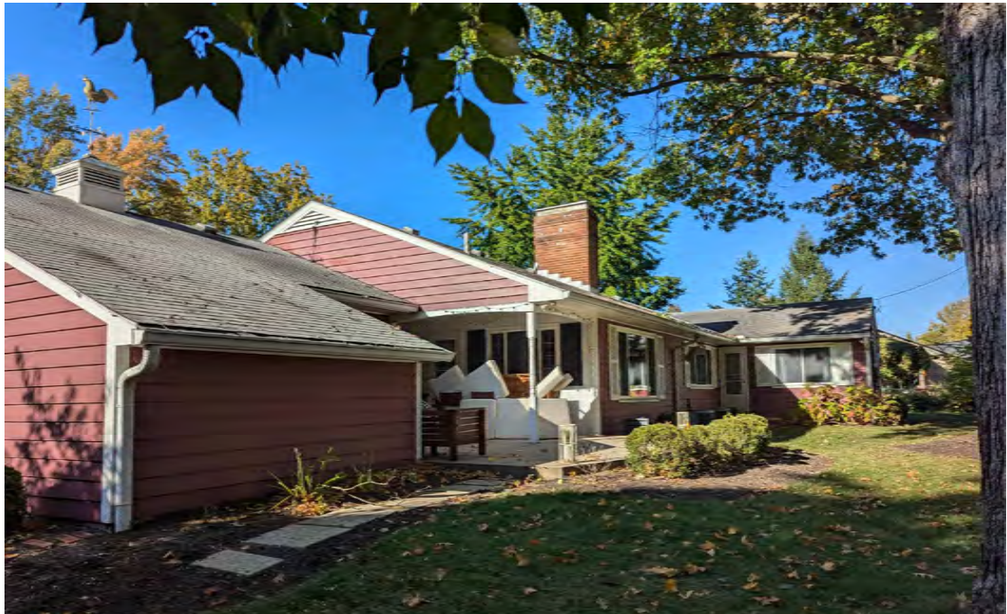
3 Existing East Rear Elevation - Photo
