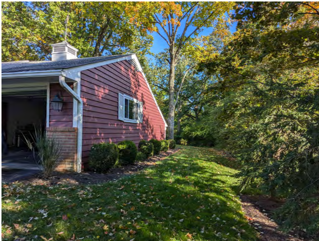
3 Existing South Side Yard - Photo
