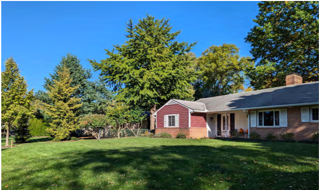
④ Existing Northwest Front Entry - Photo
