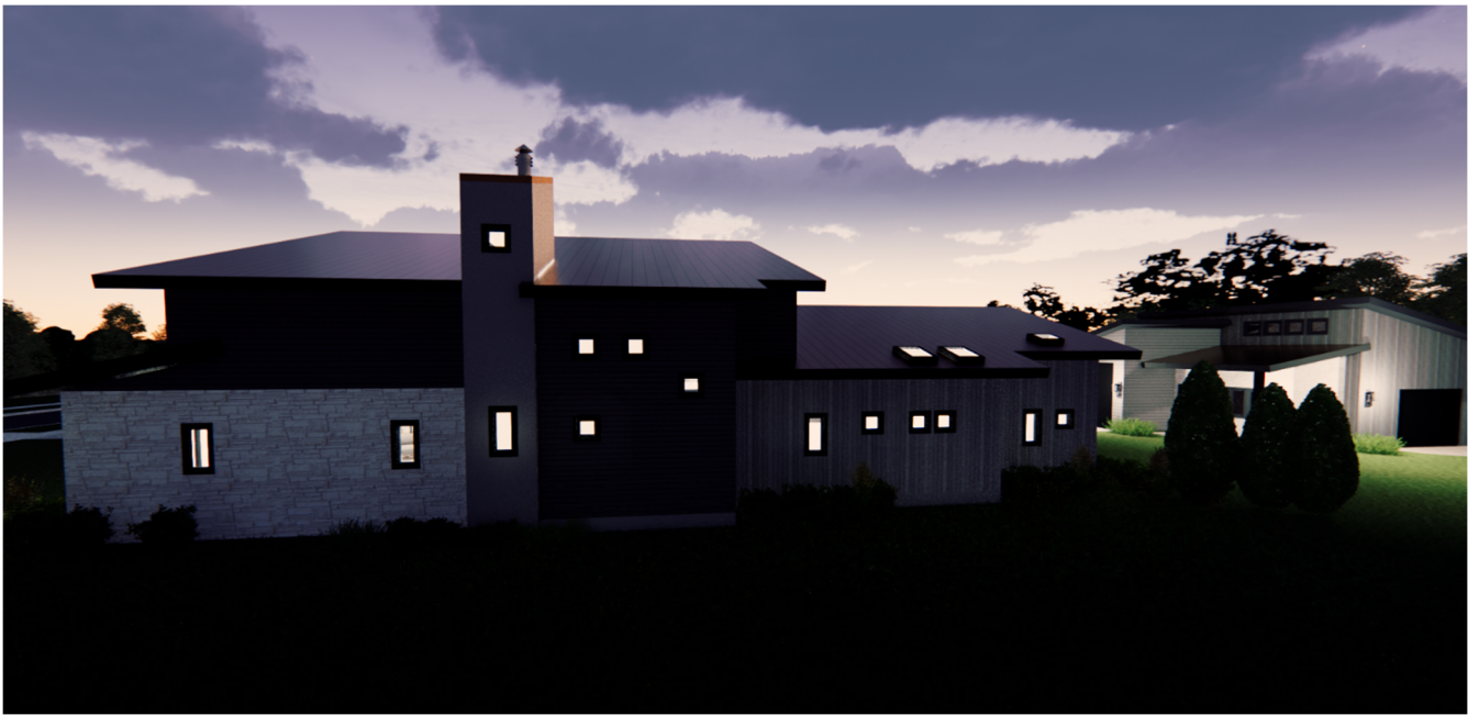
EAST SIDE VIEW LOOKING WEST - DUSK
