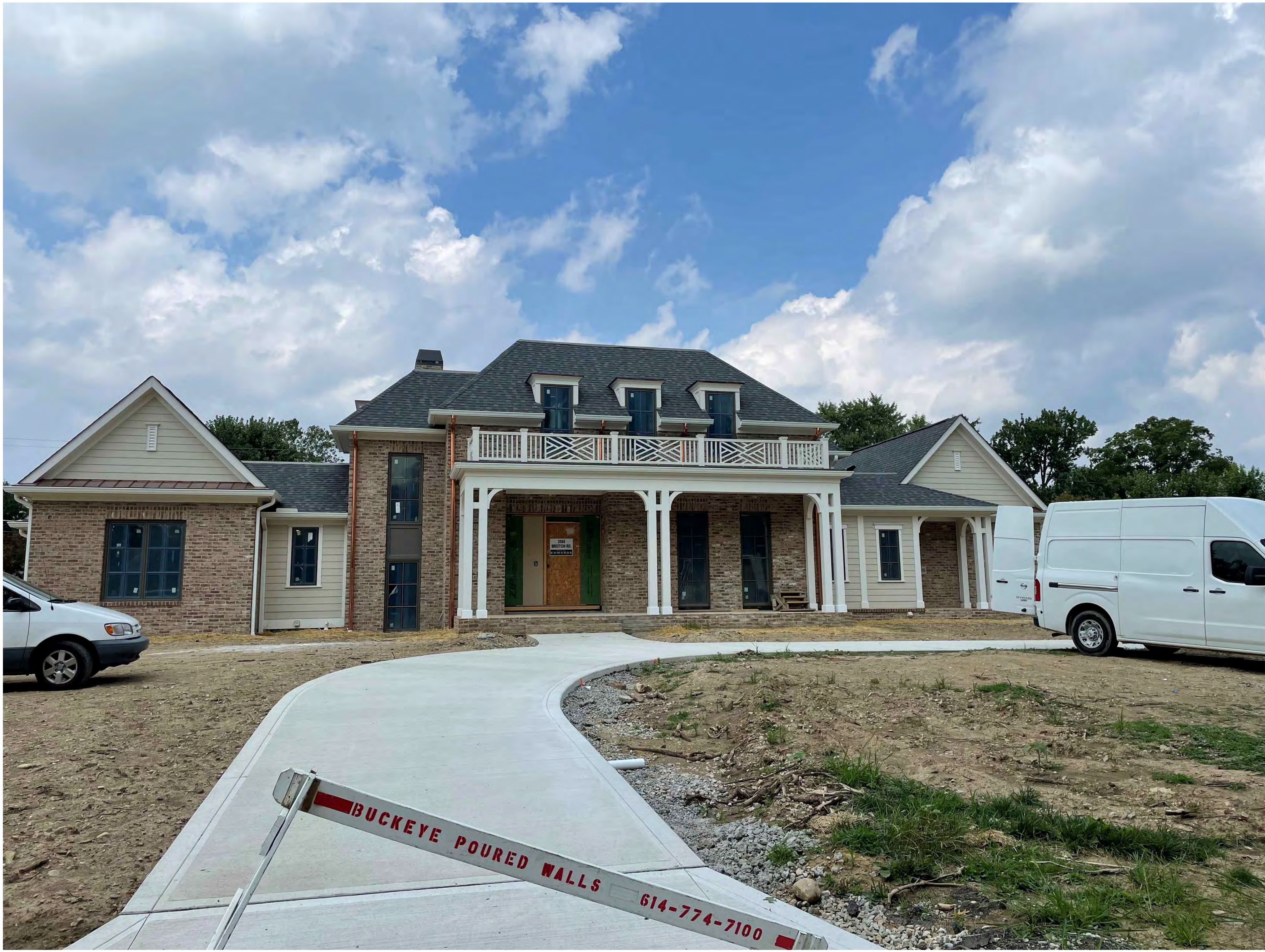
SAMPLE HOUSE PICTURES SCALE: N.T.S. LOOKING NORTH
