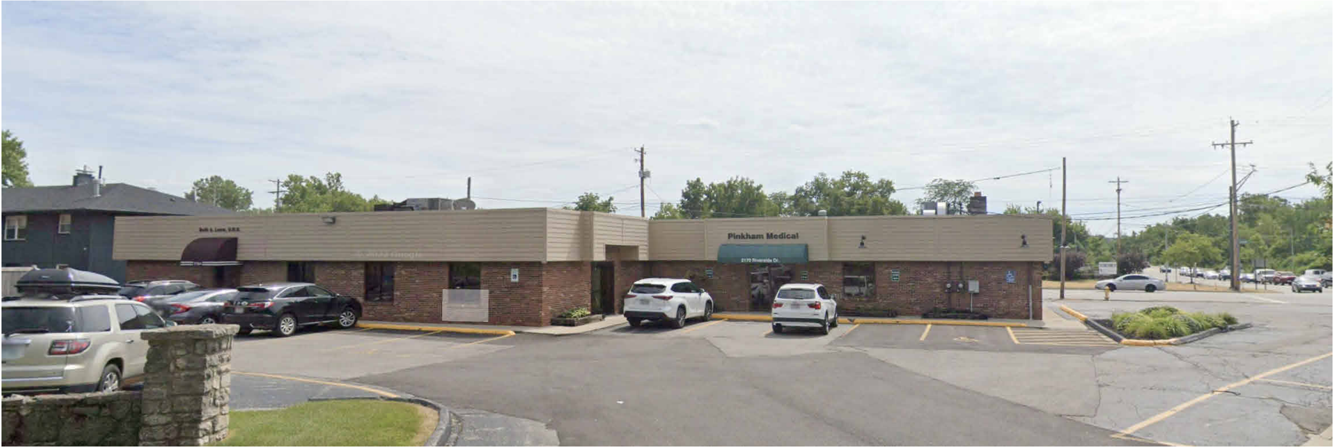
EXISTING VIEW OF EAST ELEVATION
