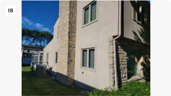
NE corner and East elevation
