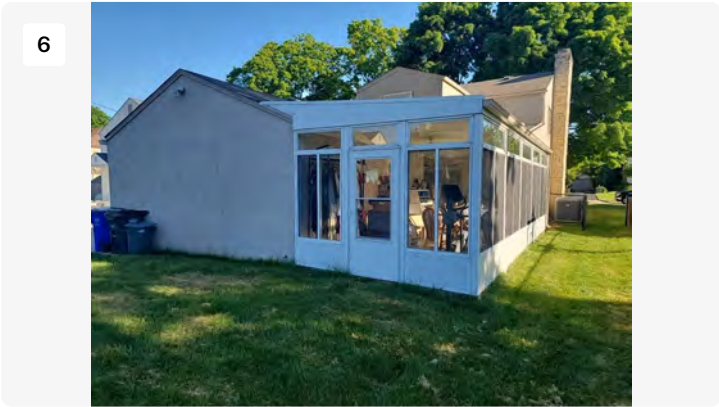
South and east elevations
