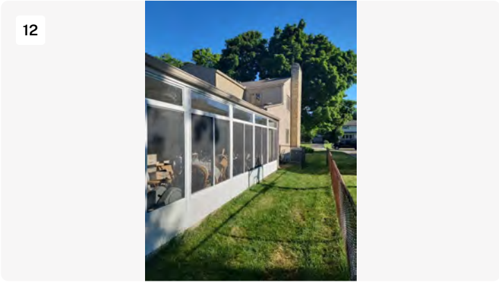
East side of house
