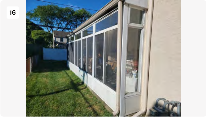
Existing patio enclosure
