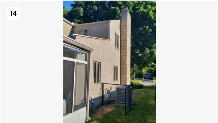
2' fireplace bump out from main house, matches porch enclosure.
