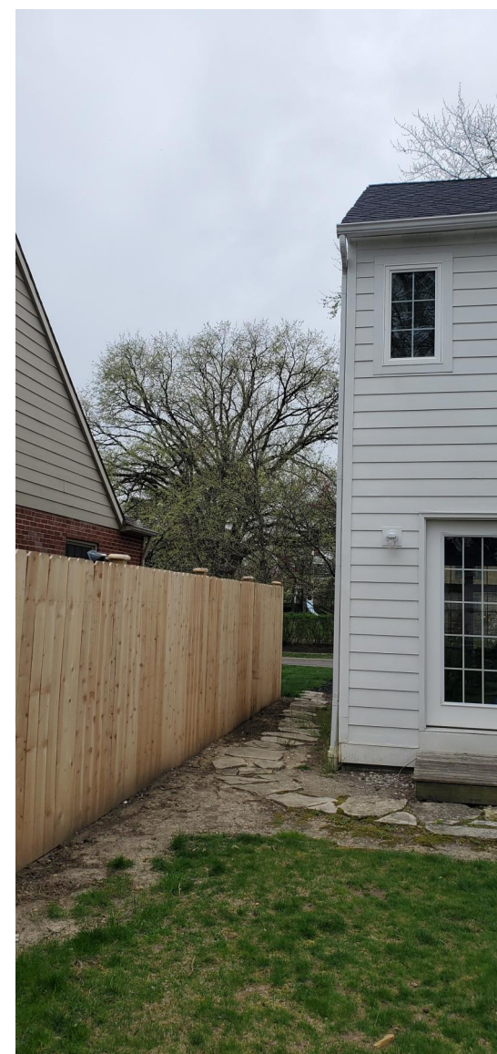
EXISTING SIDE YARD FROM REAR
