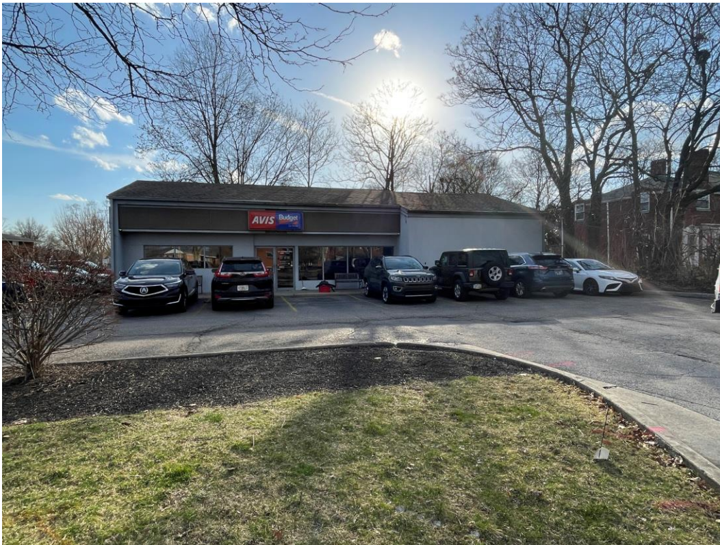
Figure 6: Existing Northwest Boulevard elevation
