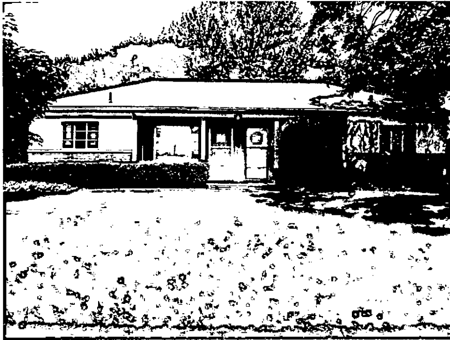
Figure 1 – Existing one-story apartment building fronting on Tremont Road
