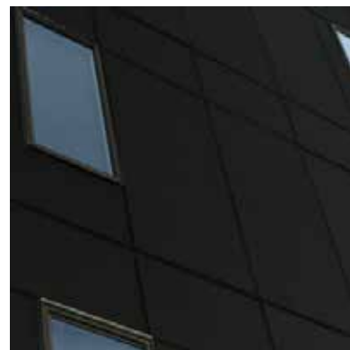
2 FIBER CEMENT HARDIE PAINTED
